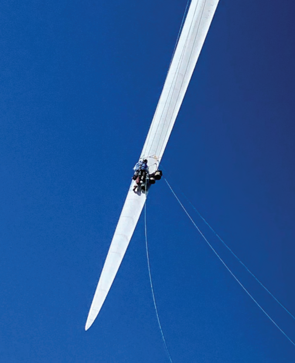
A technician repairs a blade at the Block Island Wind Farm. Photo: Andrew Ahern
