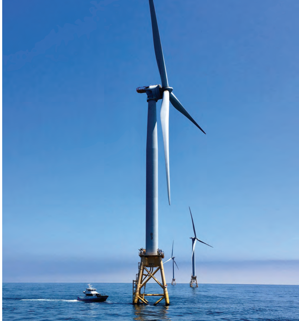
Block Island Wind Farm. Photo: Amber Hewett
