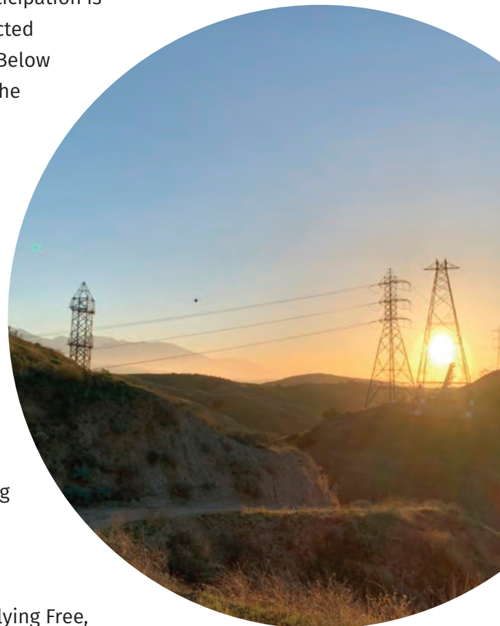
Morongo Transmission LLC
